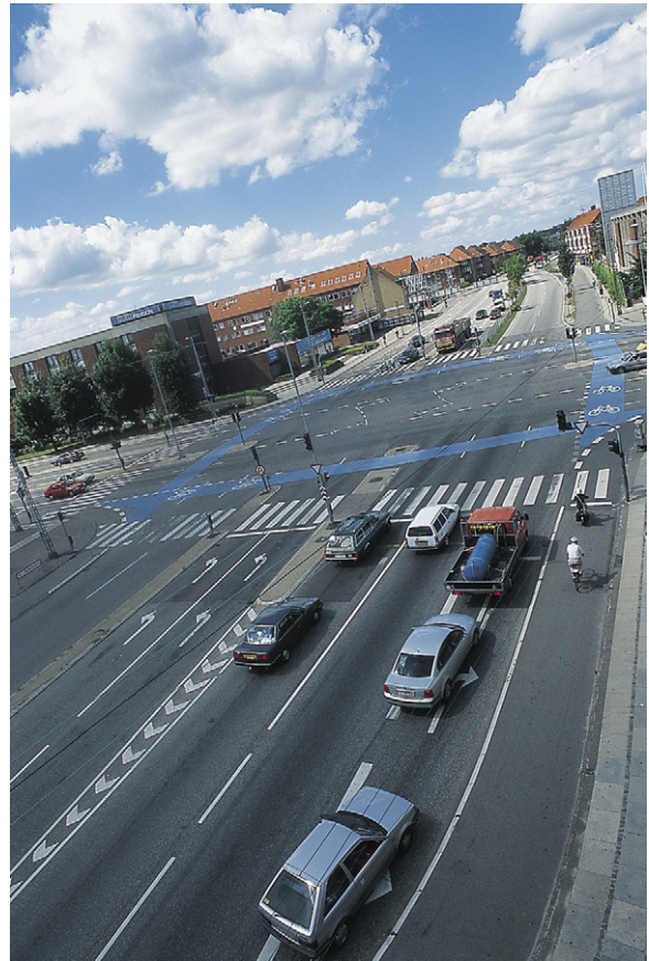
Fig. 1. Photo of signalised junction in Copenhagen with four blue cycle crossings.
